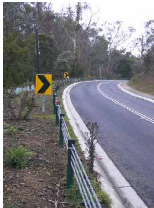
Figure 20 Four rope wire rope barrier
